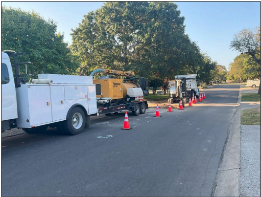
Water Distribution team excavates site in preparation for repairing water main
