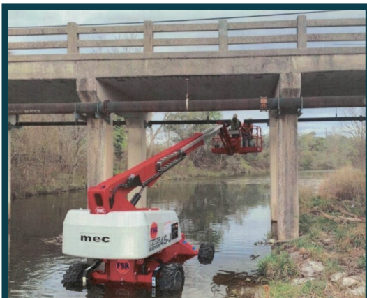
Repairing lines under bridge
