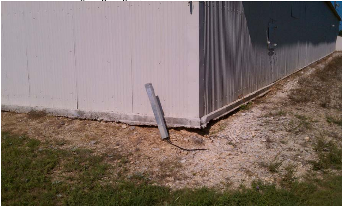
Opposing wing of Bldg. 18, notice the thinness of the foundation
