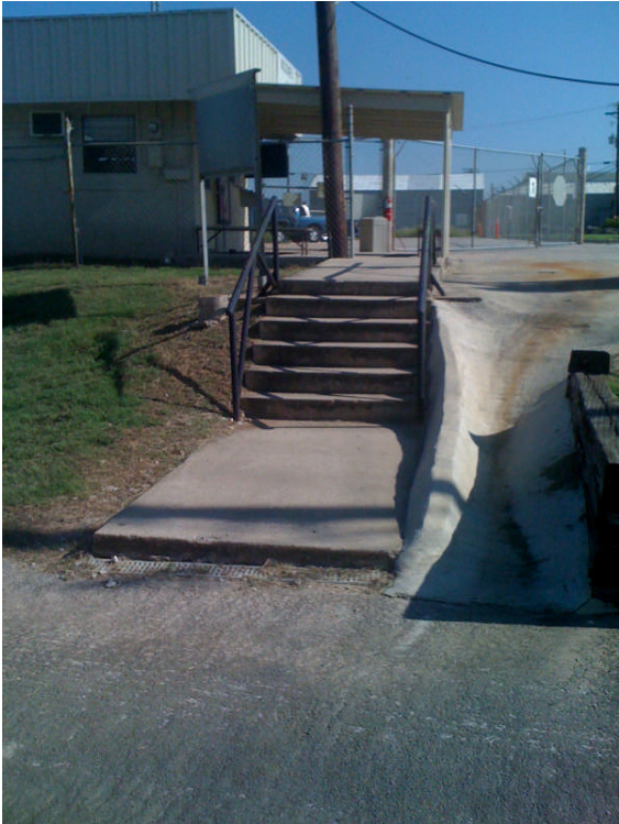
Stair transition from parking to main building (No ramp present)
