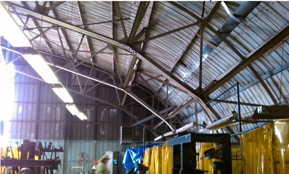
Barrel Vault Trusses above Machine Shop
