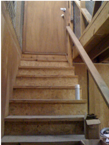
Example of non compliant stair railing
