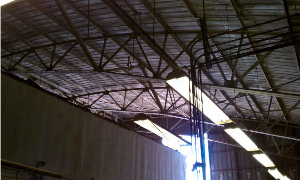
Barrel Vault Trusses above Machine Shop
