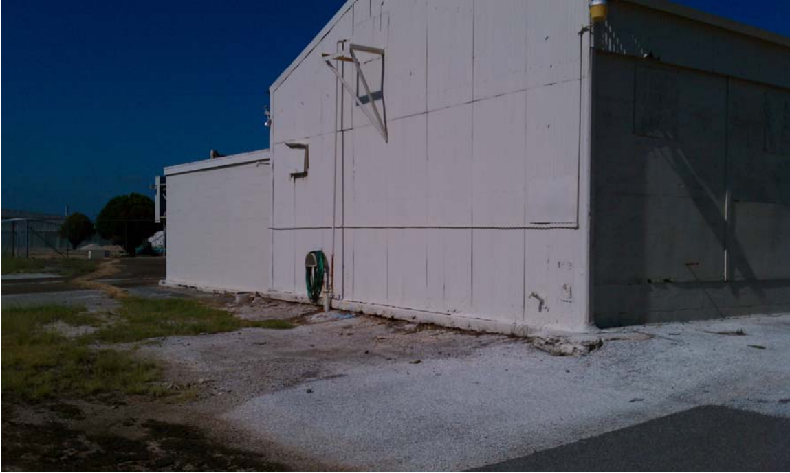
Testing wing Bldg 18, Notice the thinness of the foundation.
