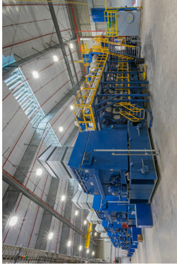
Similar natural gas-fired reciprocating internal combustion engine plant owned and operated by Denton Municipal Electric.
