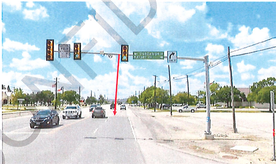
Figure 2: Facing West on Highway 27 (April 2023) One camera mounted to the traffic light arm capturing two lanes.
