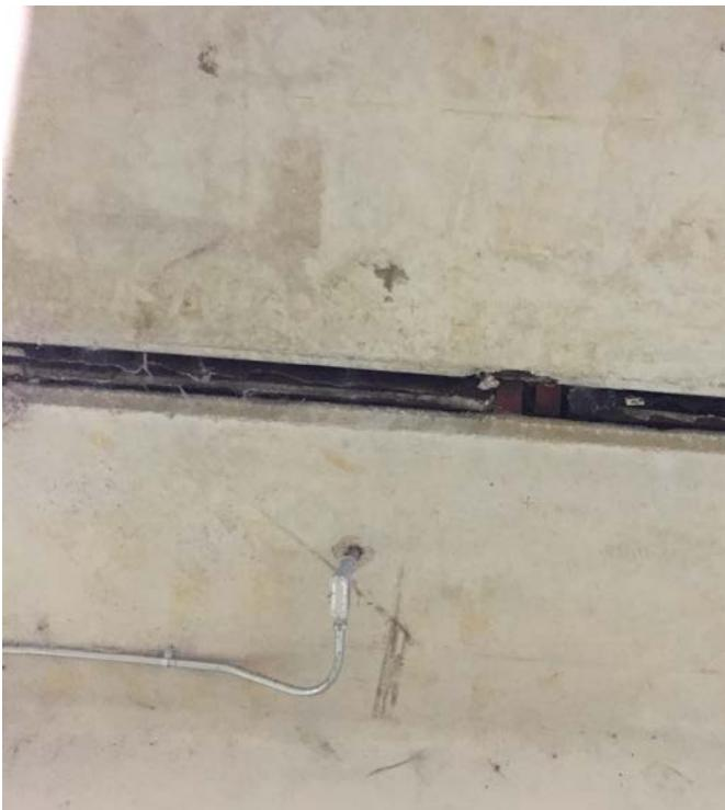
Typical underside of failed expansion joint with evidence of previous repair
