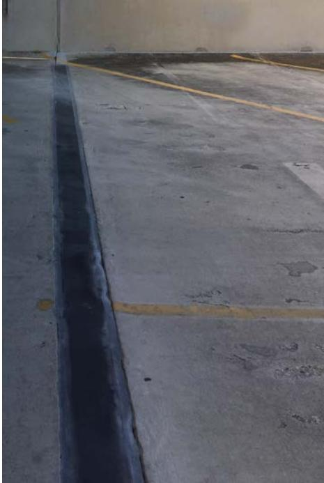
Typical failed expansion joint. Topping damage visible to right.
