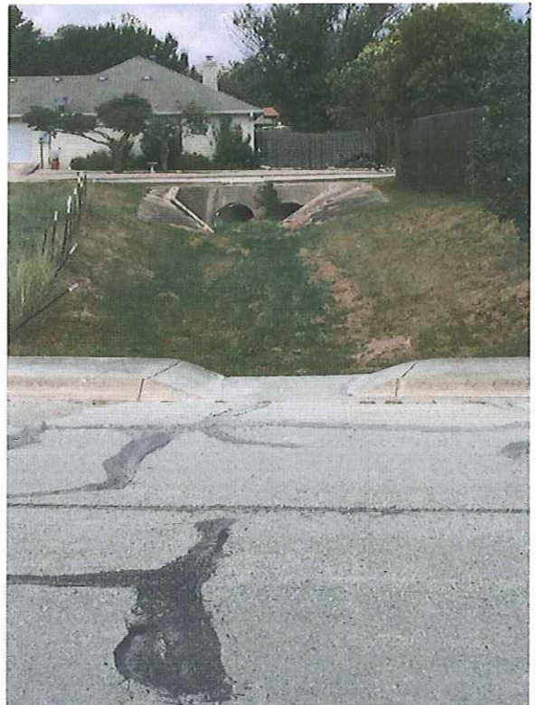
Village Glen drainage channel headwall where flow is discharged to culverts under Coronado Drive. This is not maintained by the City of Kerrville.
